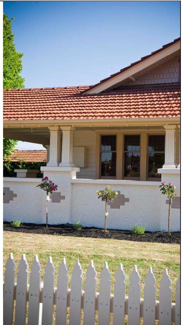
Roof tiles cleaned and coated Feature brickwork
