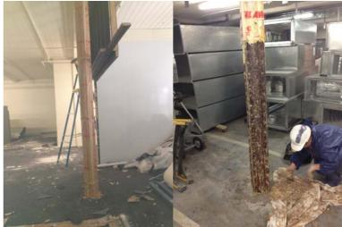
Poles are coated in stripper and covered in paper until paint is activated. Right pic shows lead paint removal.
